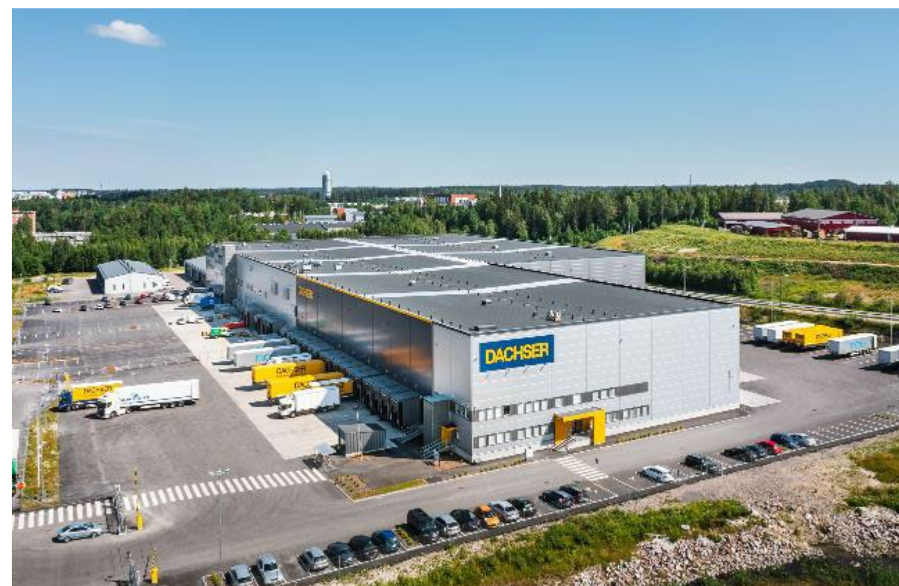
Logistics Terminal, NREP, Kerava
