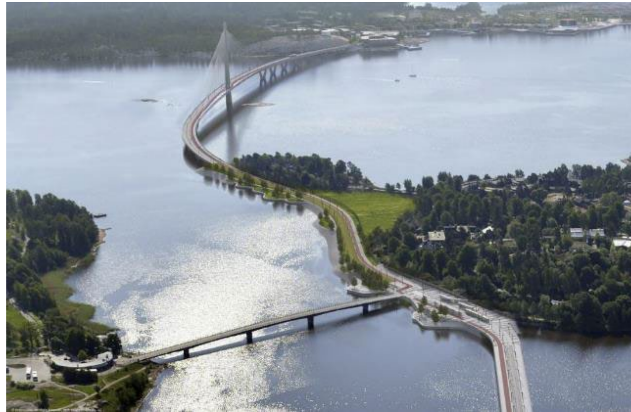
The Crown Bridges, City of Helsinki, Helsinki
