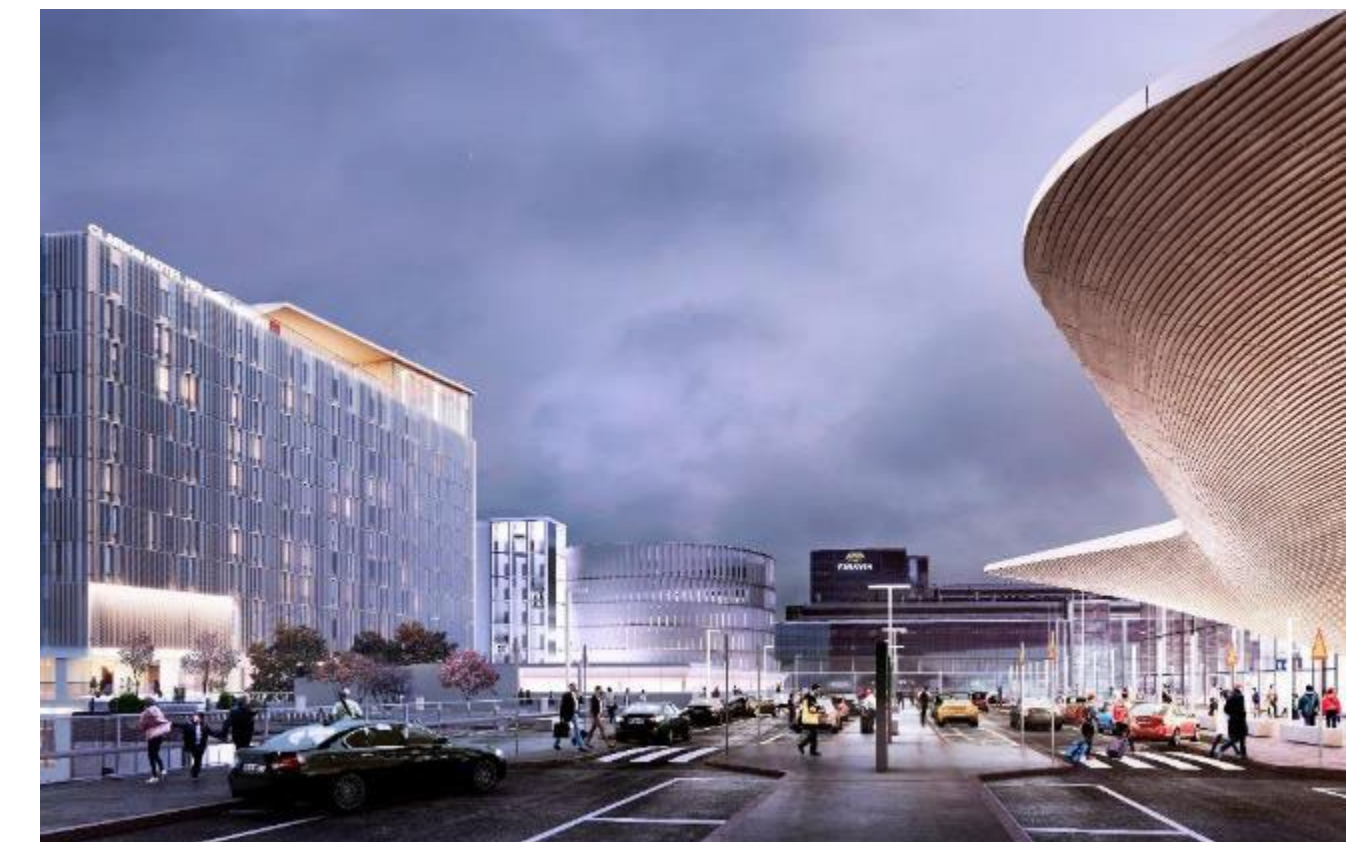
Airport hotel, AVIA Real Estate, Vantaa
