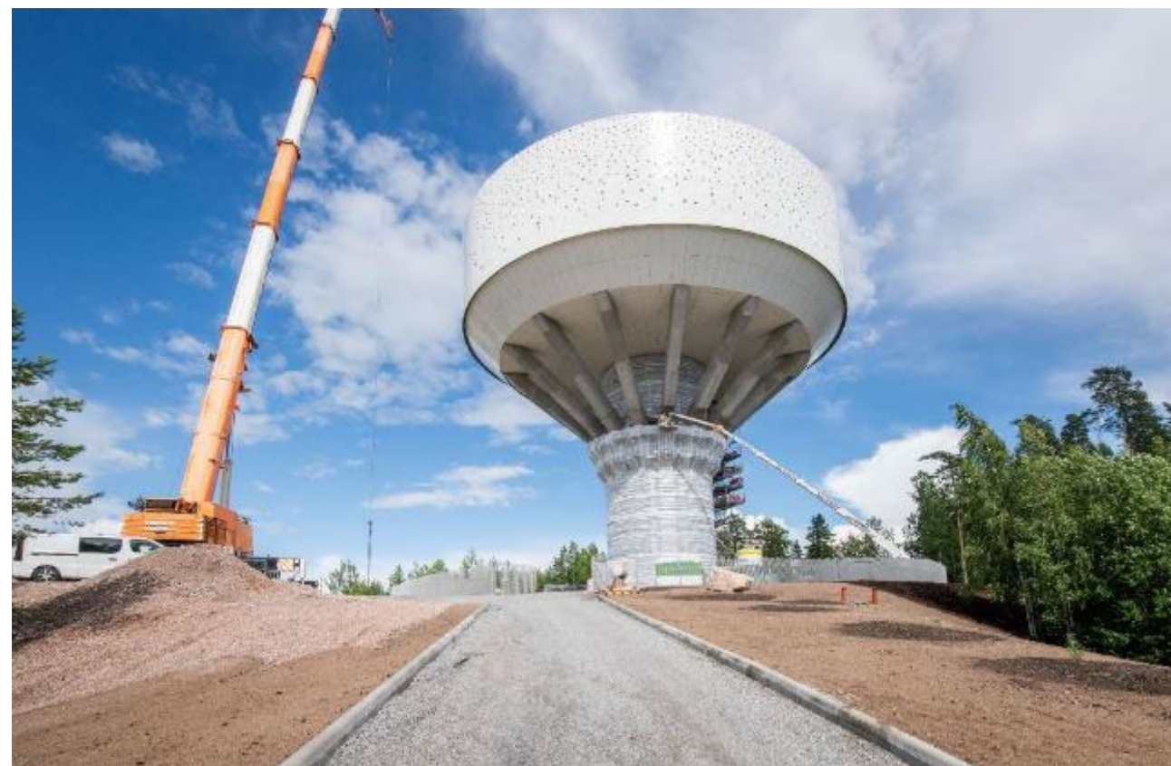
The water tower in Hiekkaharju, HSY, Vantaa
