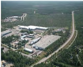
Sievi, Finland Electronics and mechanics Personnel 310 Floor area 26 000 m2
